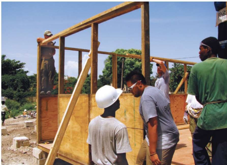
Break Away students help workers in Haiti build a new structure for Fois et Joie, a program of Jesuit Refugee Services.
