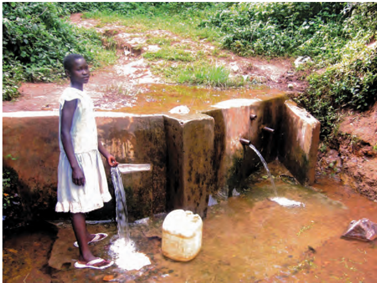
A girl in Kenya's Kisii District draws water from a local spring that has been protected through concrete sealing.
